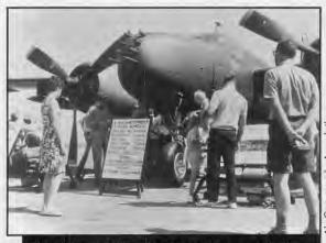
The eight .50 caliber heavy machine guns in this A-26A Counter Invader's nose could put out nearly 6,000 rounds per minute. It reigned as the most effective truck-killer on the Ho Chi Minh Trail until the arrival of another prop aircraft — the AC-130 gunship.
